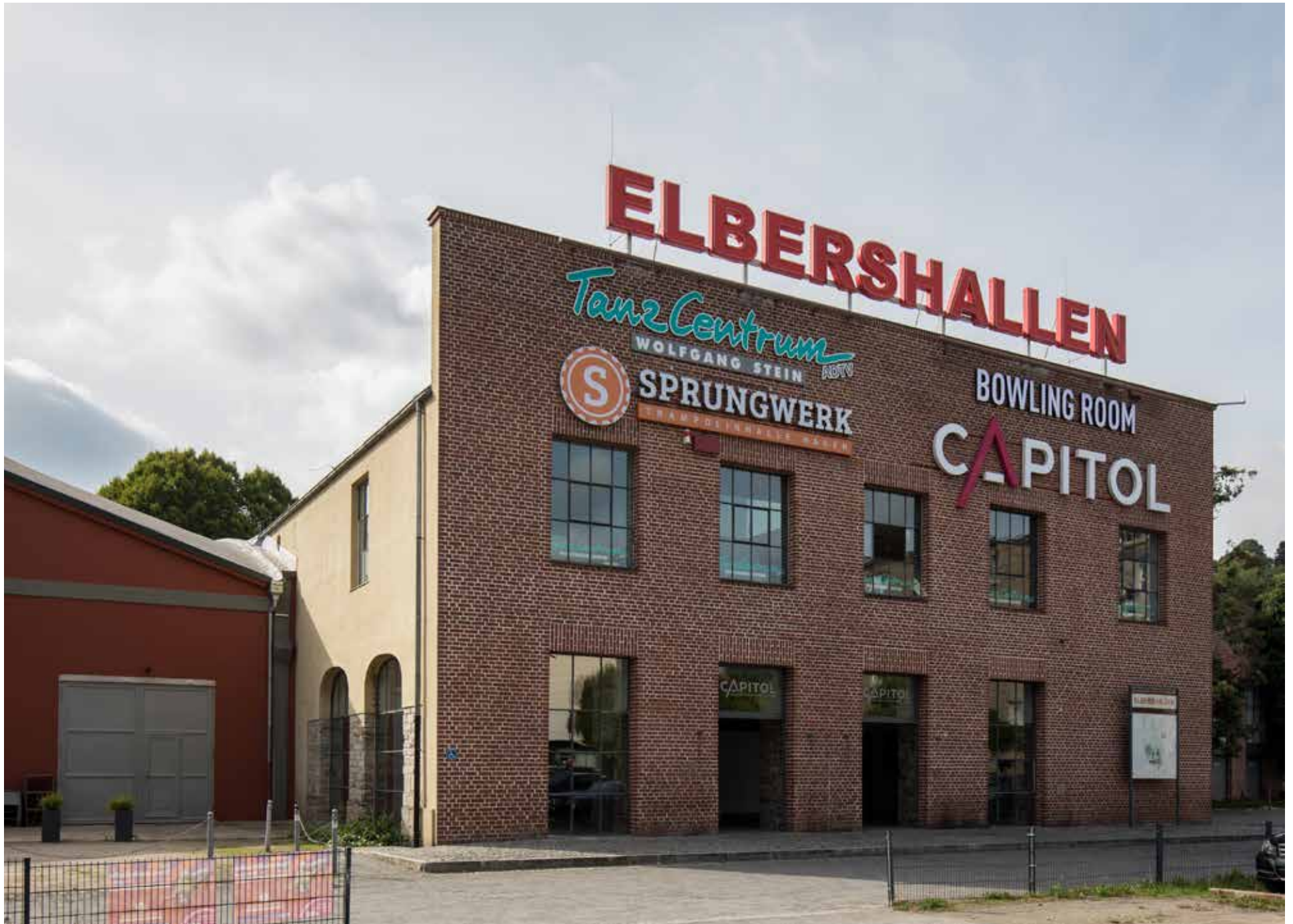
Bowling Room Hagen - Hagen, Germany - 15 lanes - Boutique
